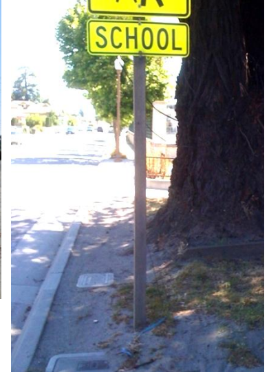
Figure 12: Sidewalk missing near school zone
