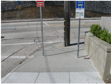
Figure 1: Obstructions in crosswalk
