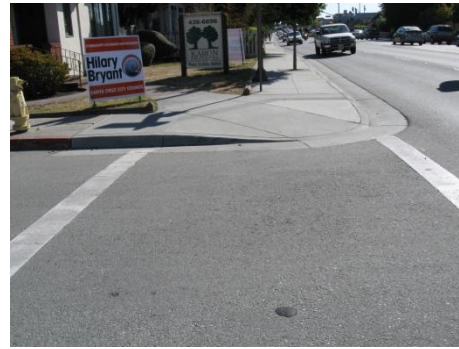
Figure 2: Curb cuts on the diagonal lead into middle of street
